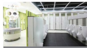
The waste water reclamation and reusing system recycles about 50 tons of water per day, and about 120 tons of underground water is saved by using urinals that do not require water.
